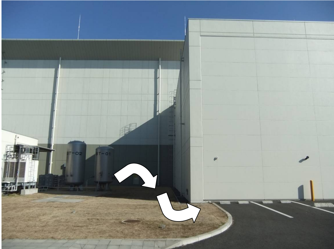
Road on the west side of MLF and detour for people on foot or bikes (indicated by arrows)(2)
